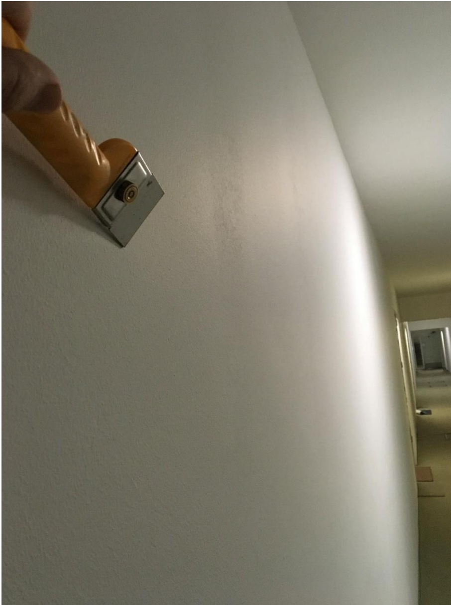
Fig 2, Walls affected by critical lighting, where the light is not hitting the wall sections this appears to be smooth with an even finish
